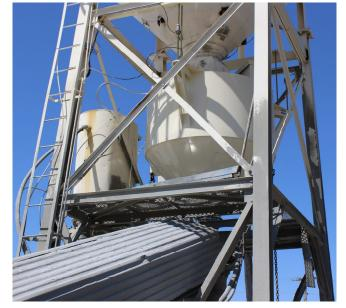
**SOLUTION:** 5yd<sup>3</sup> cement batcher was replaced with a 10yd<sup>3</sup> cement batcher which eliminated double batching.
